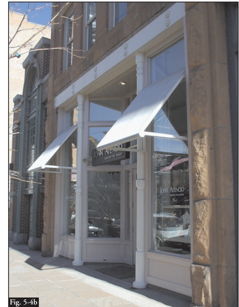
Fig. 5-4 Awnings are an inexpensive way to add shade, animation, and weather protection to building fronts.
